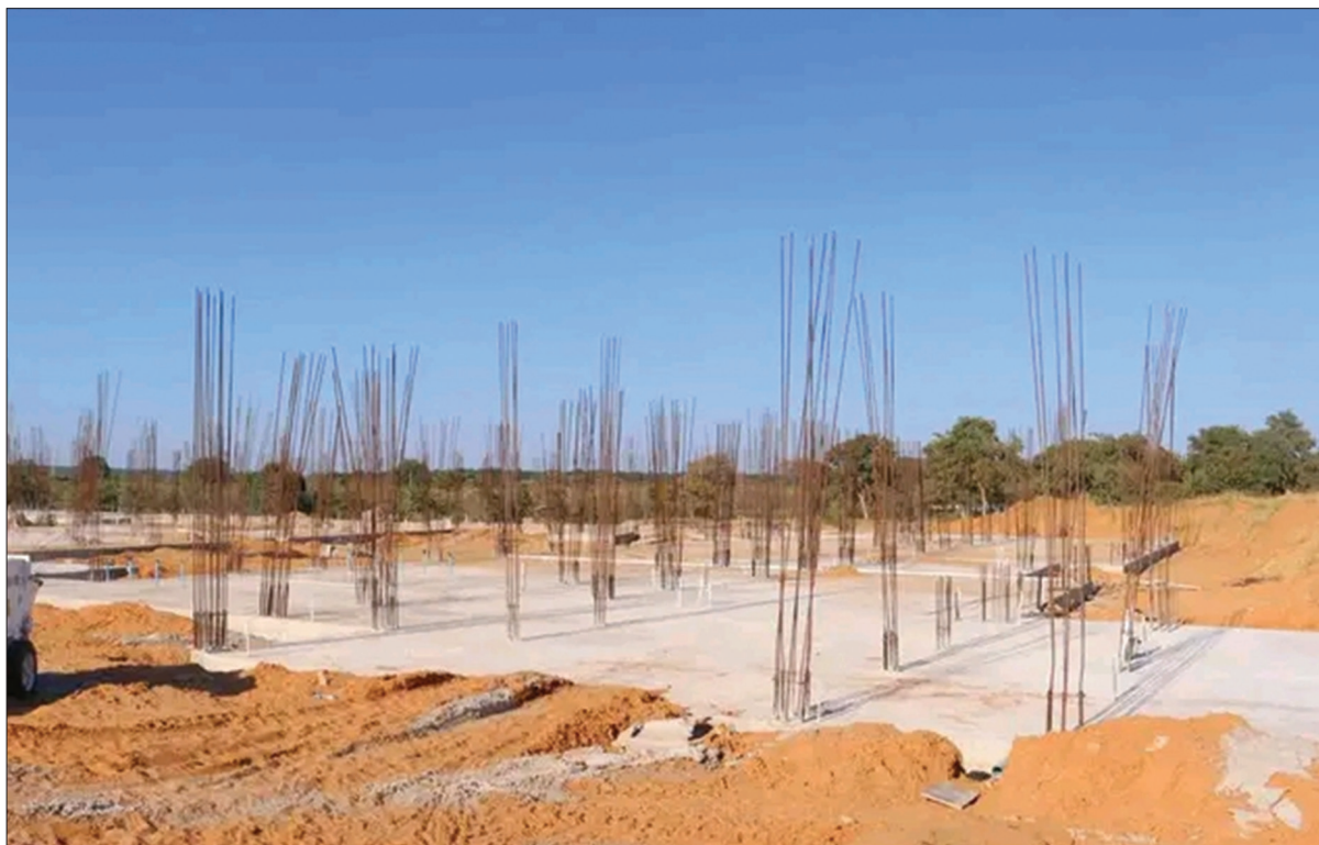
The Technovation Centre currently under construction on campus.
